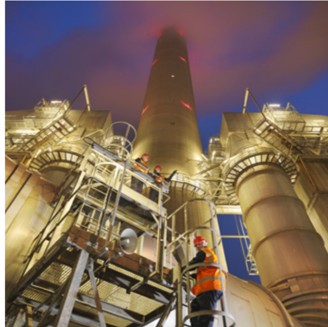
In many fields of industry, processes and systems need to operate without downtimes – even when upgrading PLCs. Migration systems offer the perfect solution.
