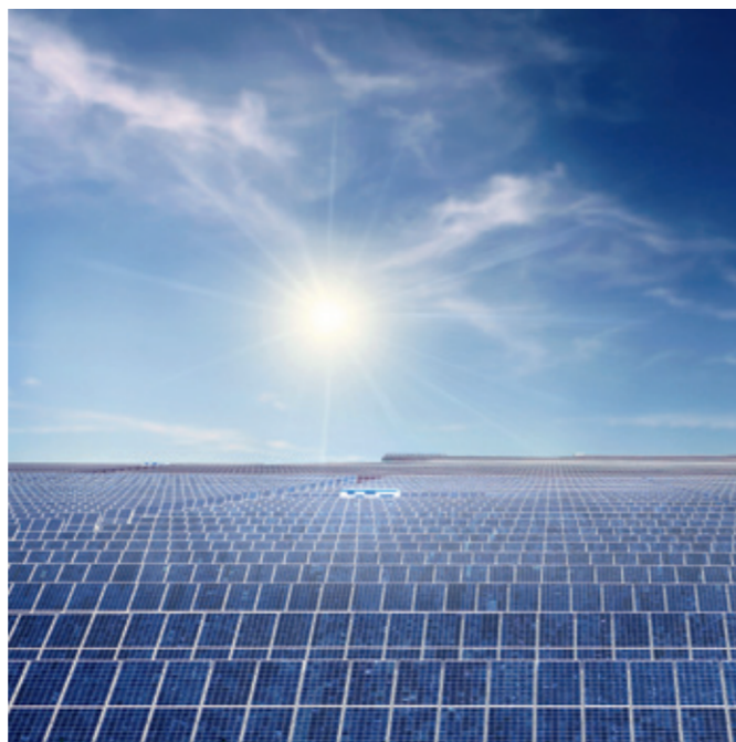
Today, return on investment is crucial for the success of a photovoltaic system. The cost aspect will become even more important in the future too due to growing competitive pressure.
