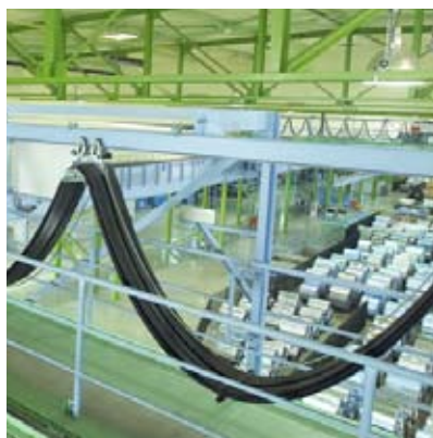
Energy and data transmission on a steel-mill-crane
