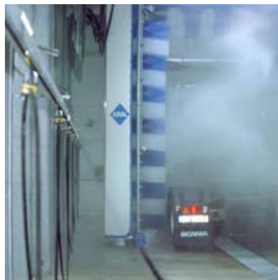
Hose-transportation in a truck washing facility
