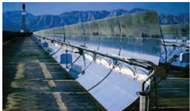
Solar-thermal parabolic trough power plant
